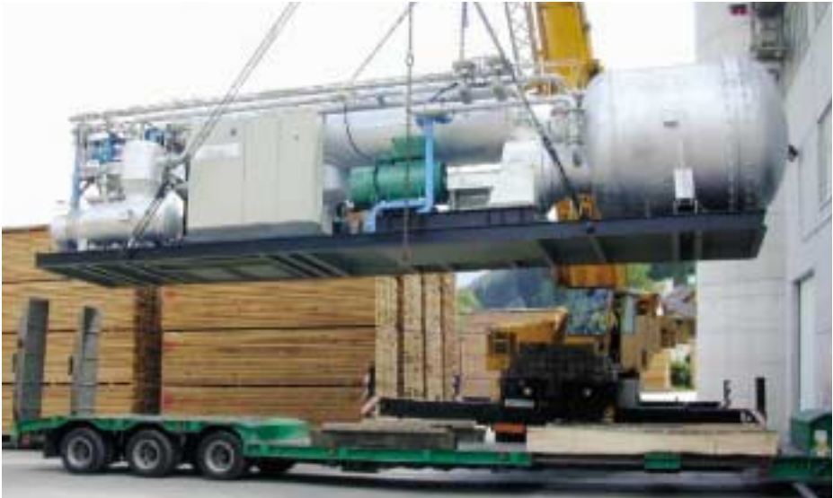
ORC-Anlage in Admont
